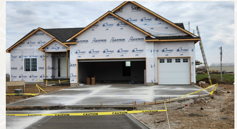
Pella: Fountain Hills New Construction
